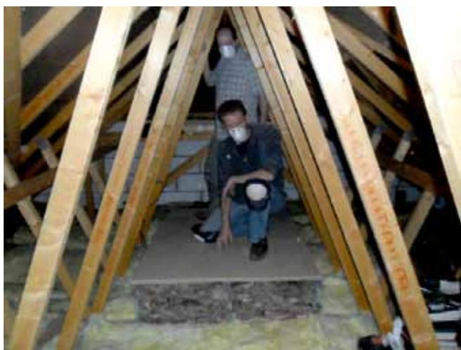
*The prototypes installed in a loft clearly illustrating that the system can support a considerable weight whilst protecting the insulation.*
